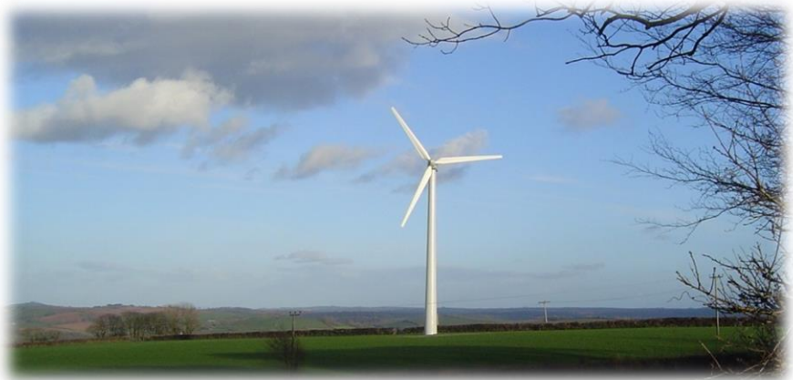
Projects like South Brent Community Energy Society's wind turbine are growing in popularity as a local response to climate change and energy prices (Credit: South Brent Community Energy Society)
