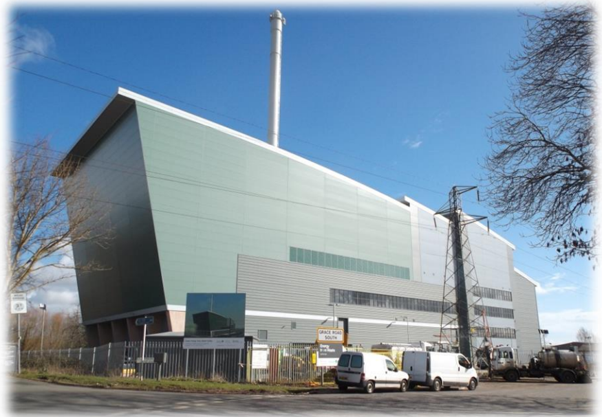
The Exeter Energy from Waste Facility received its first consignment of waste in April 2014. It treats up to 60,000 tonnes of residual, non-recyclable waste from households across Exeter, East Devon and Teignbridge.
