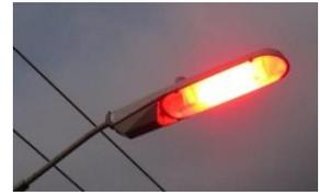
**Cons** - Only one wavelength of light is emitted (589nm - orange) resulting in low colour rendition. The lamps are often large making it difficult to direct light. Light isn't instant (they must warm up).
